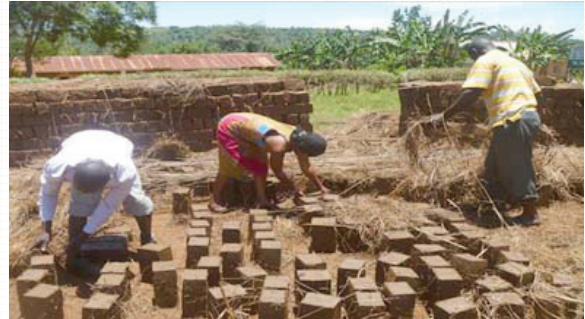
Church members at Nakateete Baptist church making bricks for church expansion.
