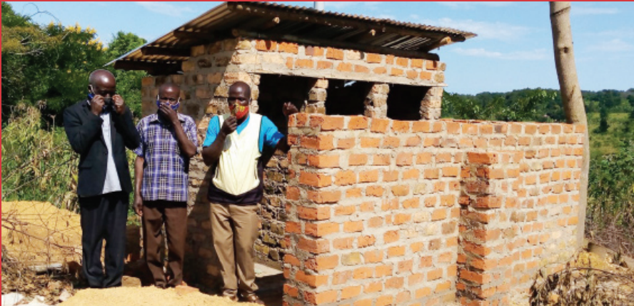
A pit latrine that was built at one of the churches as a result of community mobilisation
